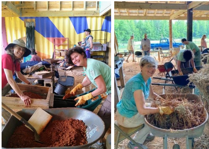
A rainy-day project—insulating a barn wall with slip straw Theresa & Amy N. sift the clay; Margaret A. is slip-strawing away
