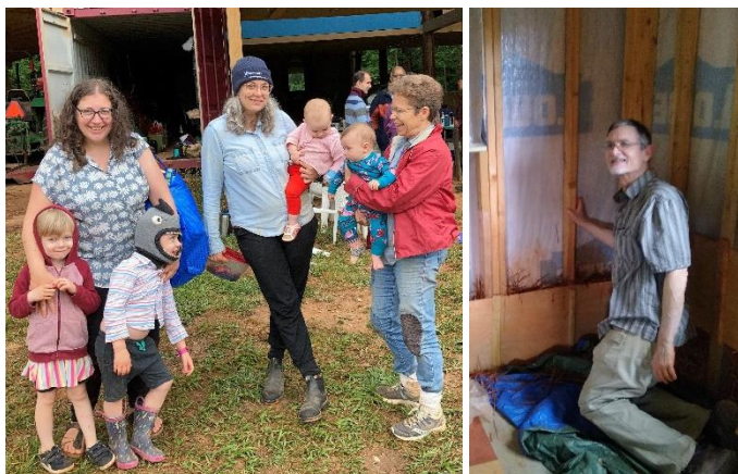
Beloved children grace the day; Bob prepares to start insulating a wall with slip straw
