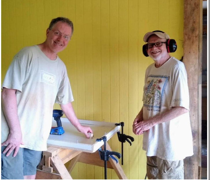
Randy and Paul conspire to create a concrete countertop
