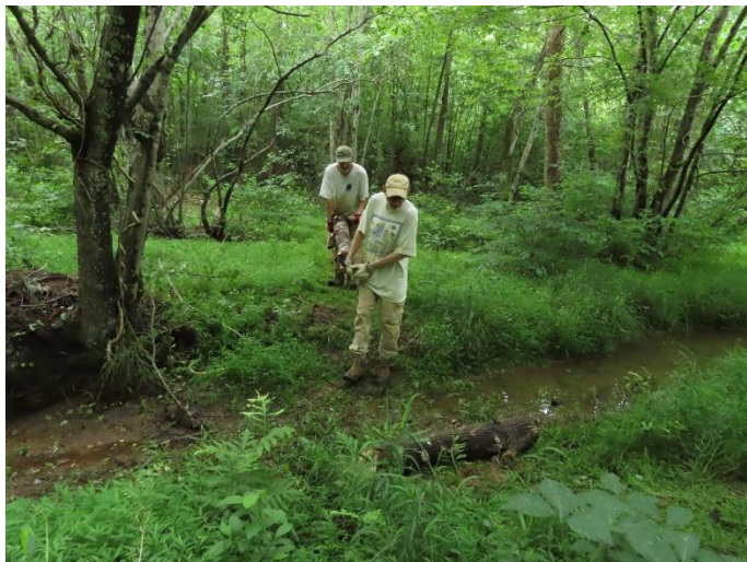
Paul and Anthony bridge a soggy gap on the new wetland crossing
