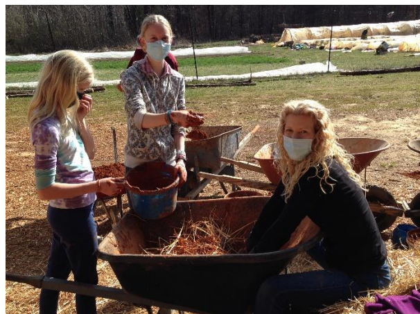
Leah and daughters prepping slip-straw insulation for the barn
