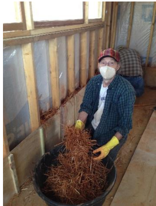
(Left) Clay, glorious clay (Right) Anthony insulates barn walls with slip-straw (straw coated with diluted clay)
