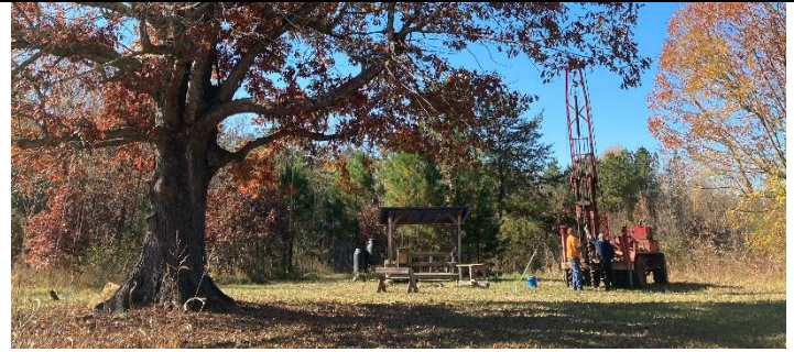
An engineering crew takes soil borings to test for our roadways
