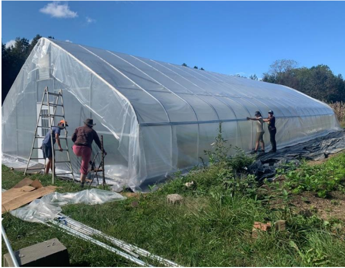
Finishing the plastic cover installation (Photo: Kai)
