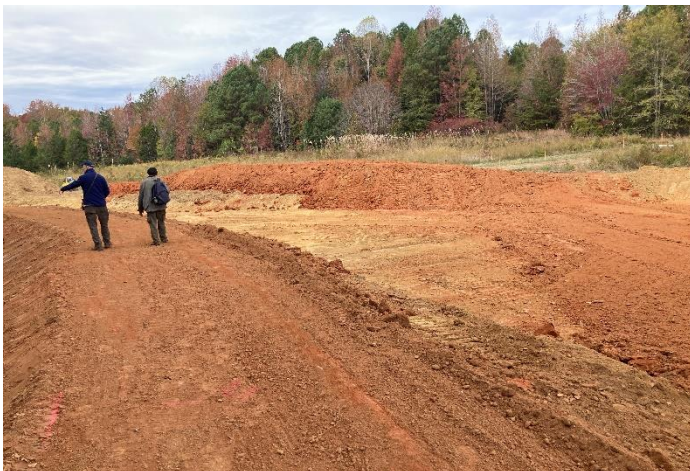
Randy & Goni witness the construction site (Photo: Hope)
