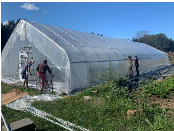
several workers secure a plastic cover onto the high tunnel (Photo: Kai)
