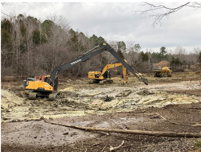
Excavators dredge and shape the pond bottom (Photo: Hope)
