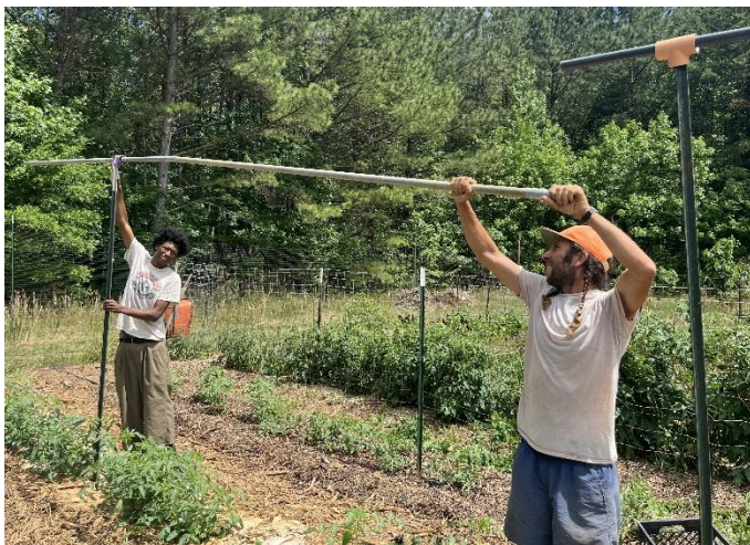
Tarase & Caleb install a sprinkler for parched crops (Photo: Kai)
